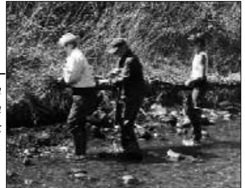
Participants in the Riparian Planting Workshop install a fascine to practice a streambank stabilization technique.
